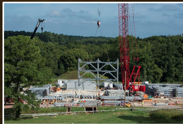
LH2 Structural Test Article (STA) Test Stand, MSFC, August 2015
